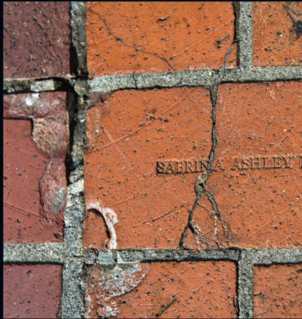
Damaged Bricks
