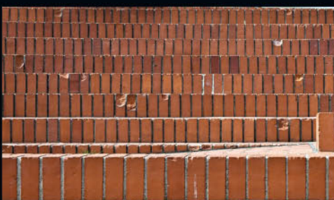
Damaged Bricks
